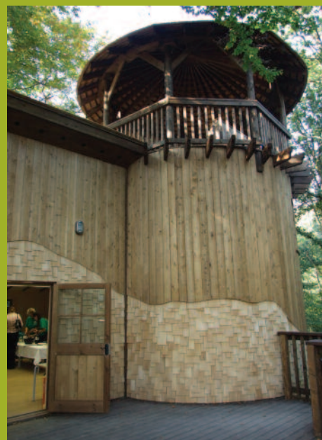
The New Forest Tree House Study Centre designed by Architecture student Samantha Sherwood
