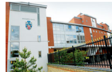
Entrance to Fenner's Building
