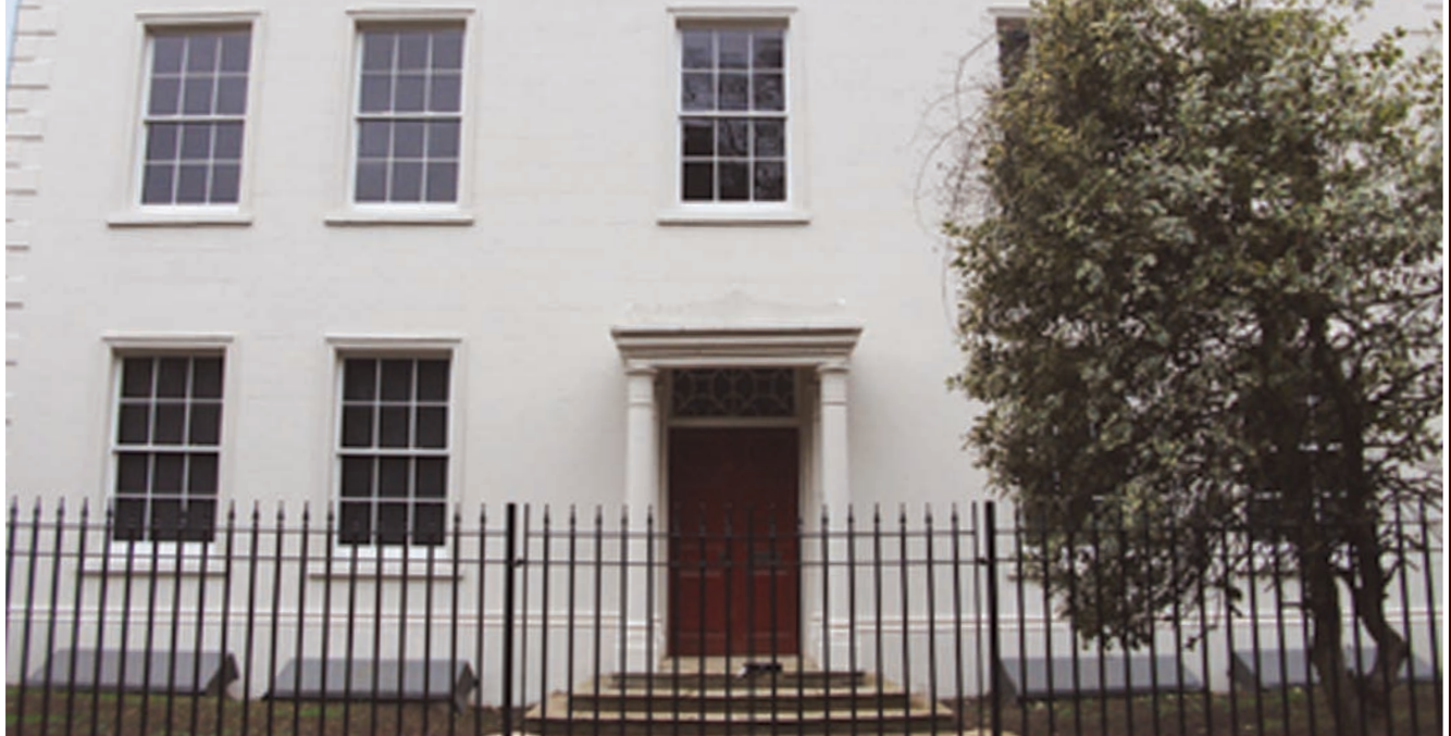
Prebend House (Phase 1 completed in 2010)
