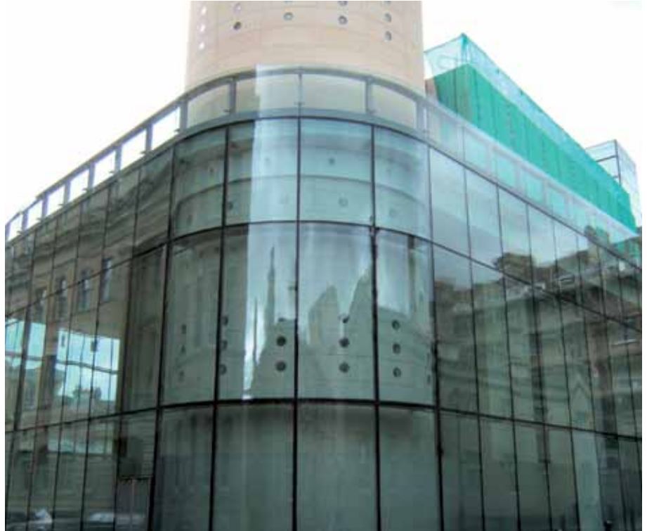
Curved point supported glass wall on the Thermae Bath Spa in Bath. The CWCT centre produced the national guidelines for risk assessment of safety of architectural glass.
