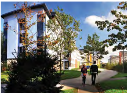
Paston House student accommodation on campus.
