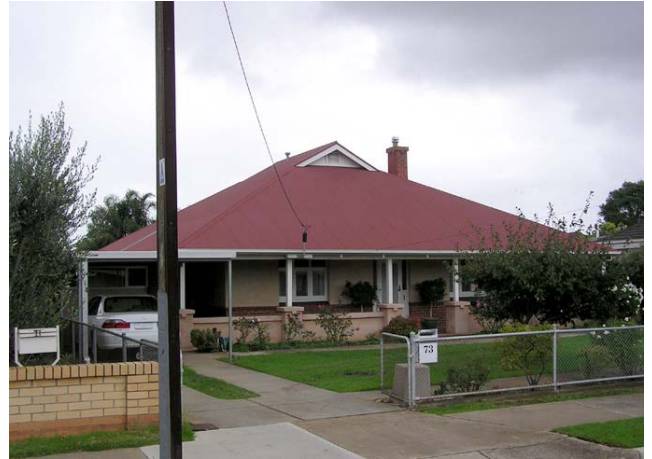
Louvre Roof 1905-1918 – gablets with louvered slats were built into the ridge cap to allow for good ventilation. Air would enter from open eaves and convection currents would force the hot air out of the gablet.
