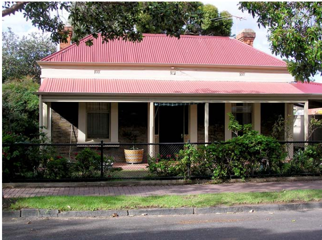
Symmetrical Cottage 1860-1915 - originally built as four room dwellings with a central hallway. Roof styles and verandah styles can vary.
