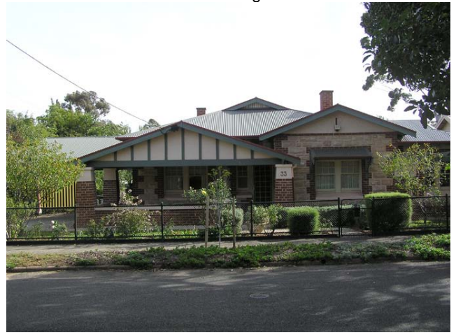
Bungalow 1916-1930 - a single story dwelling usually of rectangular shape. This style of home has a gabled front verandah.
