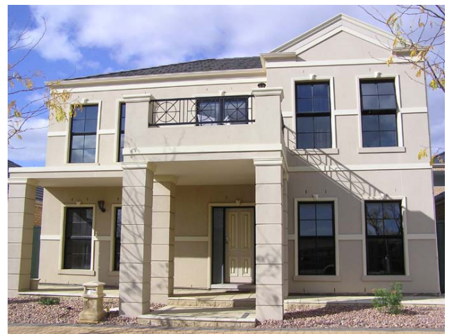
Mawson Lakes Development 1992 - present - provide a good example of today's modern building designs. These homes promote higher density developments, smaller block sizes and double story homes.
