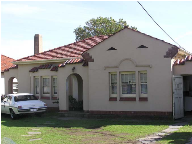
Art Deco 1934-1945 - has a steeply pitched rendered or stuccoed gable featuring front corbels in dark, often glazed brick, extended into and contrasting with the gable.
