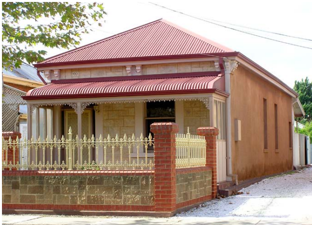
Single Fronted Cottage 1840-1915 - built from 1840 through to the early bungalow period, these homes typically have three rooms and a side hallway.
