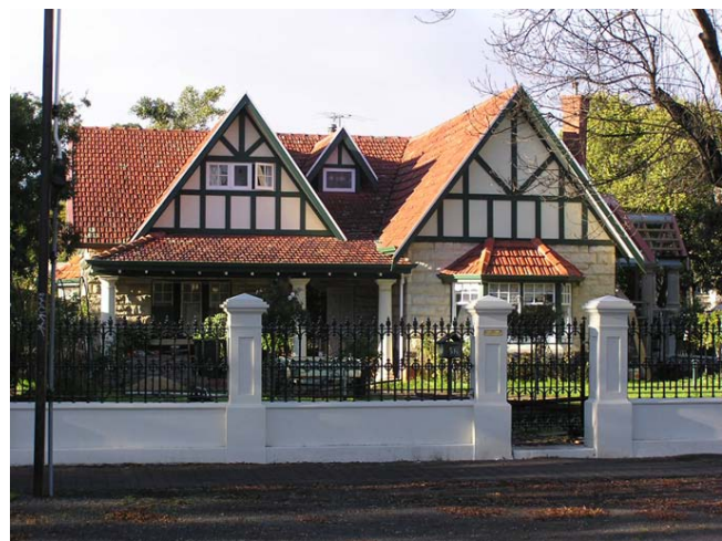
Tudor 1928-1938 - characterised by ornately decorated, steeply pitched gables. In its simplest form, this house consisted of 5 main rooms plus a sleep out under the 'lean-to'.
