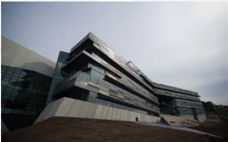
TOP ST ALBANS CAMPUS CONSISTS OF CONTEMPORARY BUILDINGS AROUND A LARGE PIAZZA AND SITS ALONGSIDE JONES CREEK AND NATIVE GRASSLANDS
